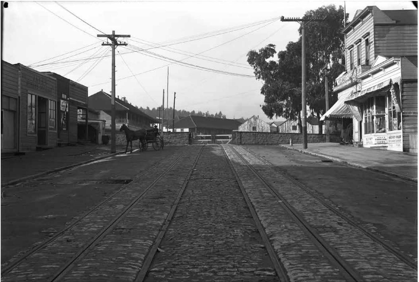
*Cable trains ran into the Presidio over this track on Greenwich Street from 1892 until 1906. Note the gap in the Presidio wall and the off-center cable slots. Photo courtesy of SFMTA.*
