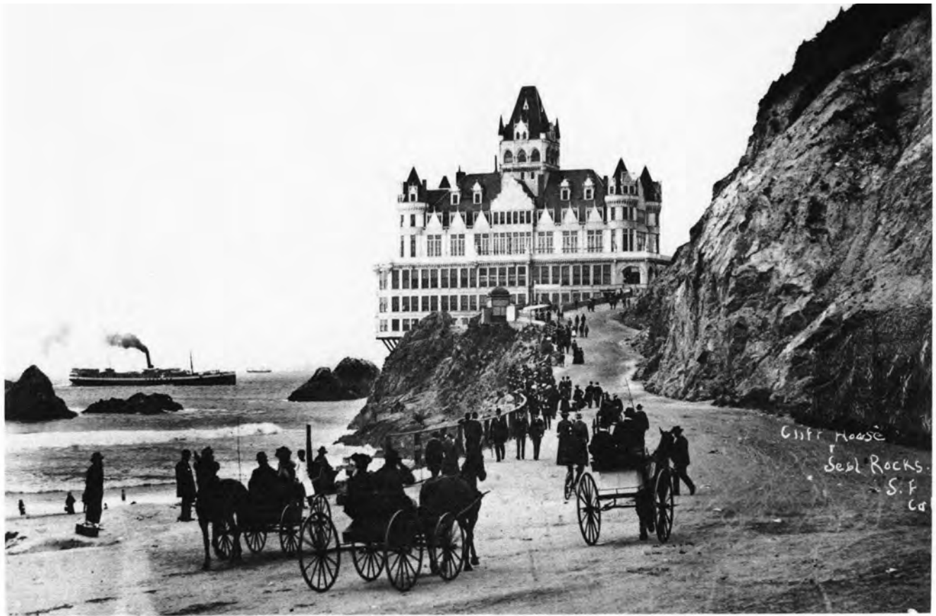
Image of the third Cliff House and Seal Rocks, 1900, from the view up Point Lobos Avenue. We see people riding carriages on the road toward the seven-story Victorian Chateau, also known as the “Gingerbread Palace” in the distance, while a steamship passes. Courtesy of a private collector.
