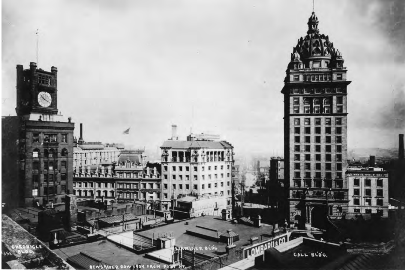
Spreckels intended the Call Building to be “the finest building ever erected for a newspaper office.” It was built on the corner of Market and Third Streets in 1897. Courtesy of the San Francisco History Center, San Francisco Public Library.
