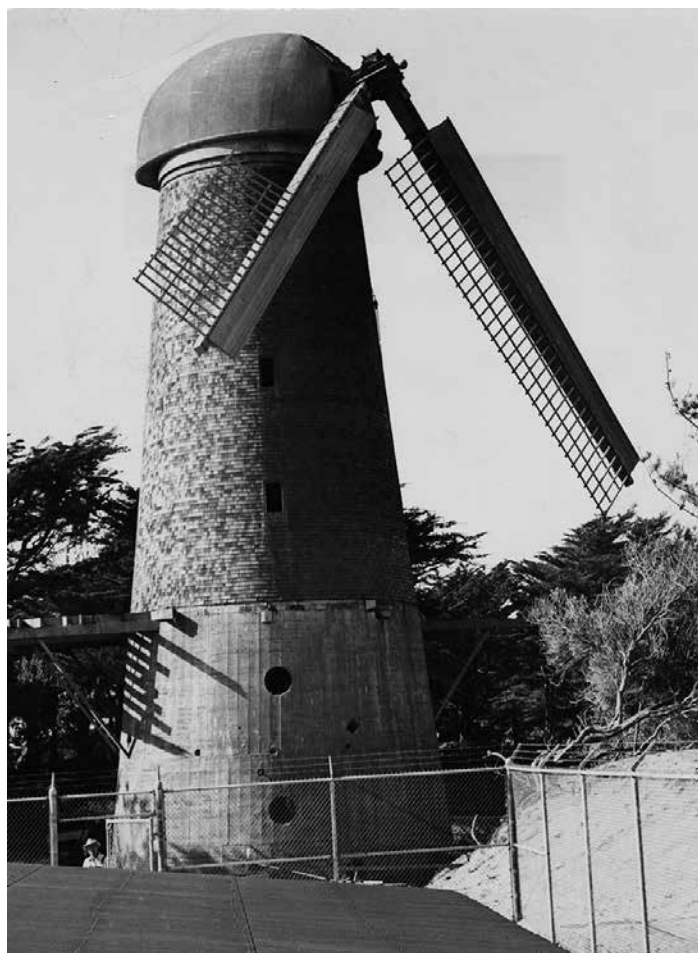
This photo shows the two remaining spars on the Murphy Windmill. Courtesy of San Francisco History Center, San Francisco Public Library.
