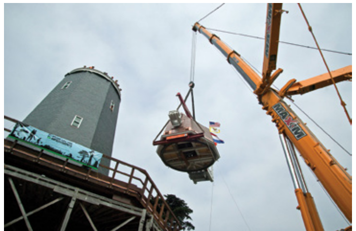
The 64-ton copper dome being lifted into place. Photo by Ron Henggeler.
