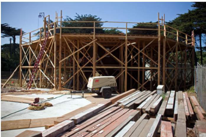
Restoration of the Murphy Windmill begins. Many of the original fir beams, visible in the foreground, were used in the restoration. Photo by Ron Henggeler.
